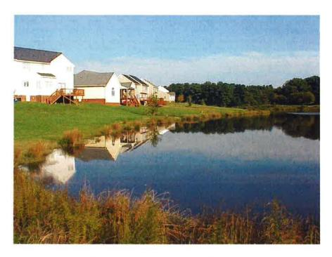
Retention basin – Note flat slopes with "rough" edge and aquatic bench provided as safety and pollutant removal features.
