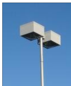
Shielded light fixture
